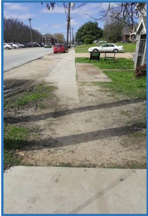
Image adapted from Jonesboro Aggie Road Walk Audit Technical Memo 2017 showing gaps in sidewalk near University.
