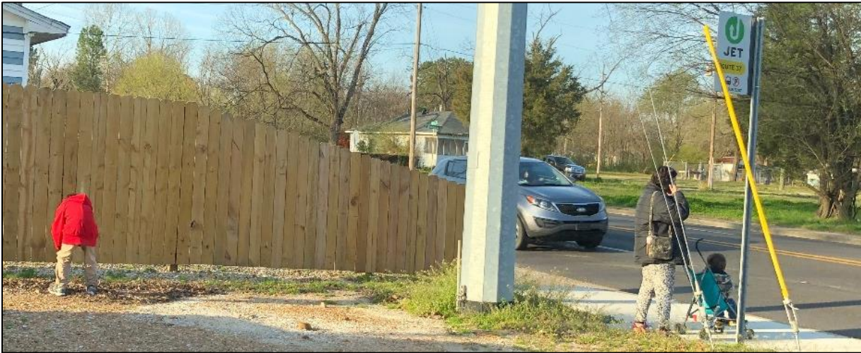
Figure 4: Lack of Accommodations at Southern Bus Stop
