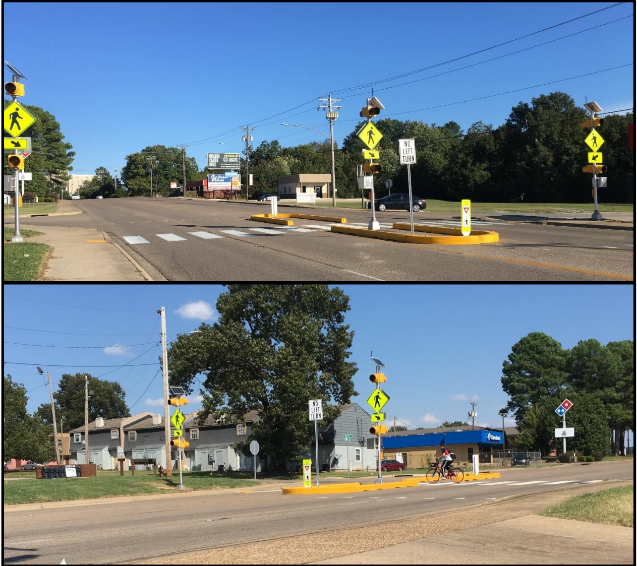
Figure 4: Temporary Pedestrian Crossing across Highway 91
