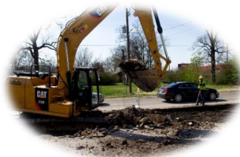
Construction of Highway 18 Overpass Photo Source: City of Jonesboro, April 2018
