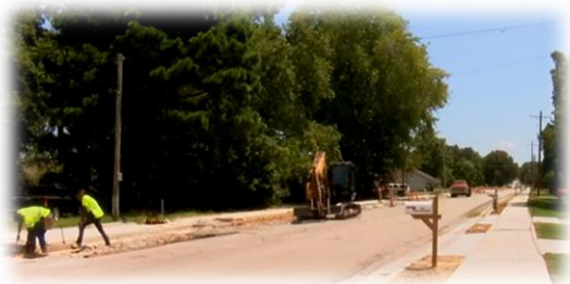
Phase II sidewalk construction on College Street in Bono
