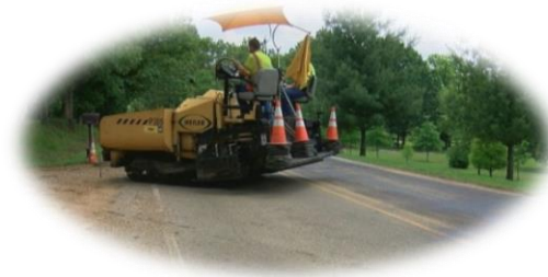
Overlay Construction on Hasbrook Rd. in Craighead County
