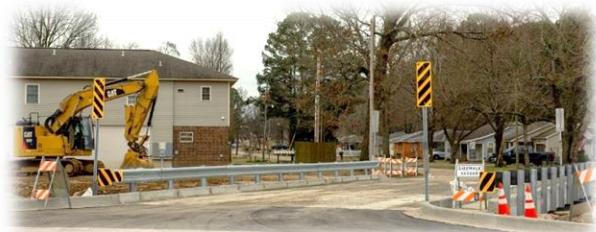
Bridge Replacement at Hester St in Jonesboro
