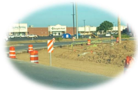
Intersection improvements at Highland Dr and Caraway Rd in Jonesboro
