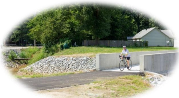
Cyclist on Turtle Creek Greenway Bridge (Phase III) in Jonesboro
